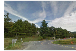
Cavendish Eastbound Begin Project MM 0.004 VT 131 and VT 103 Intersection
